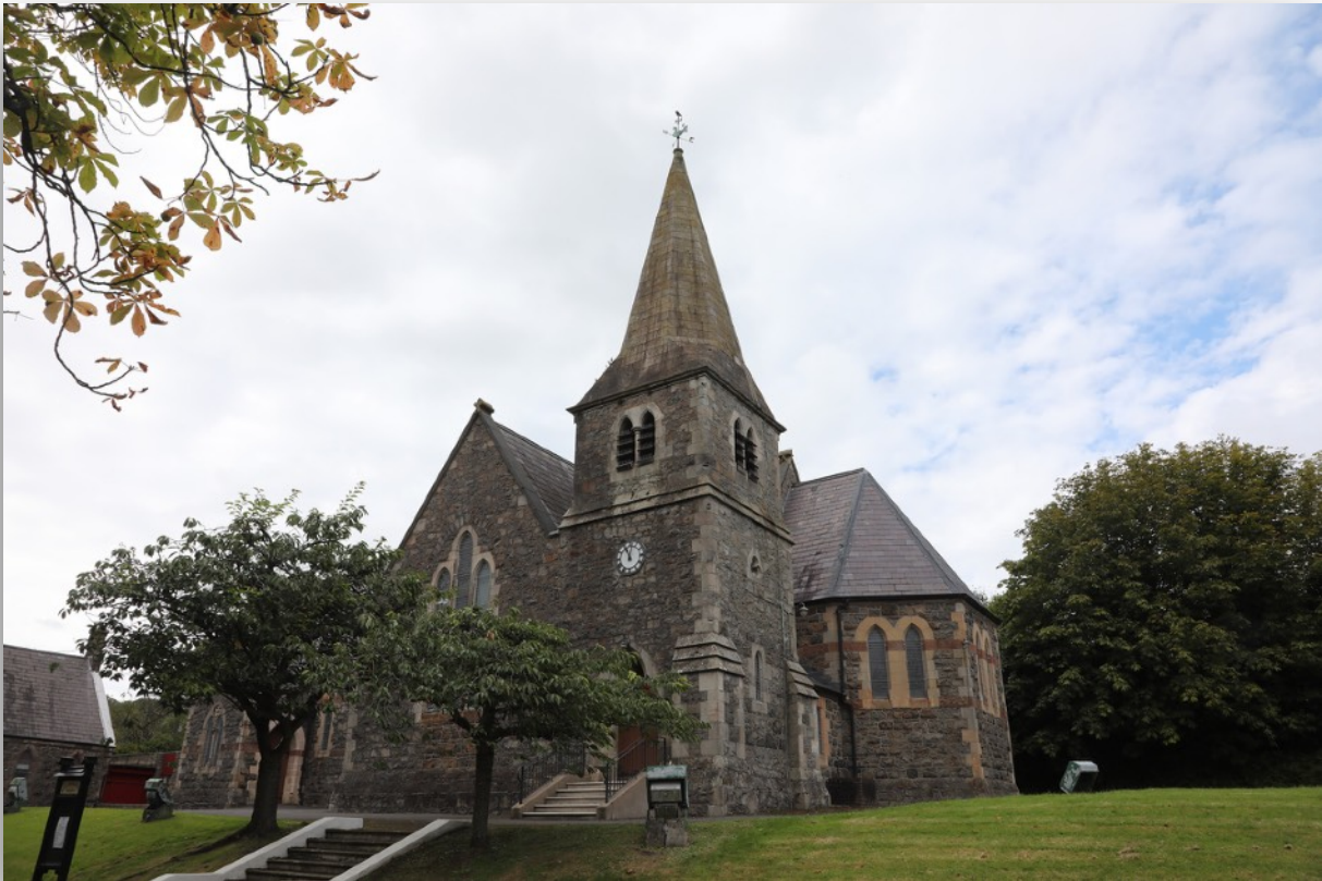
St Mark's Church, Ligonel Road, Ballysillan
